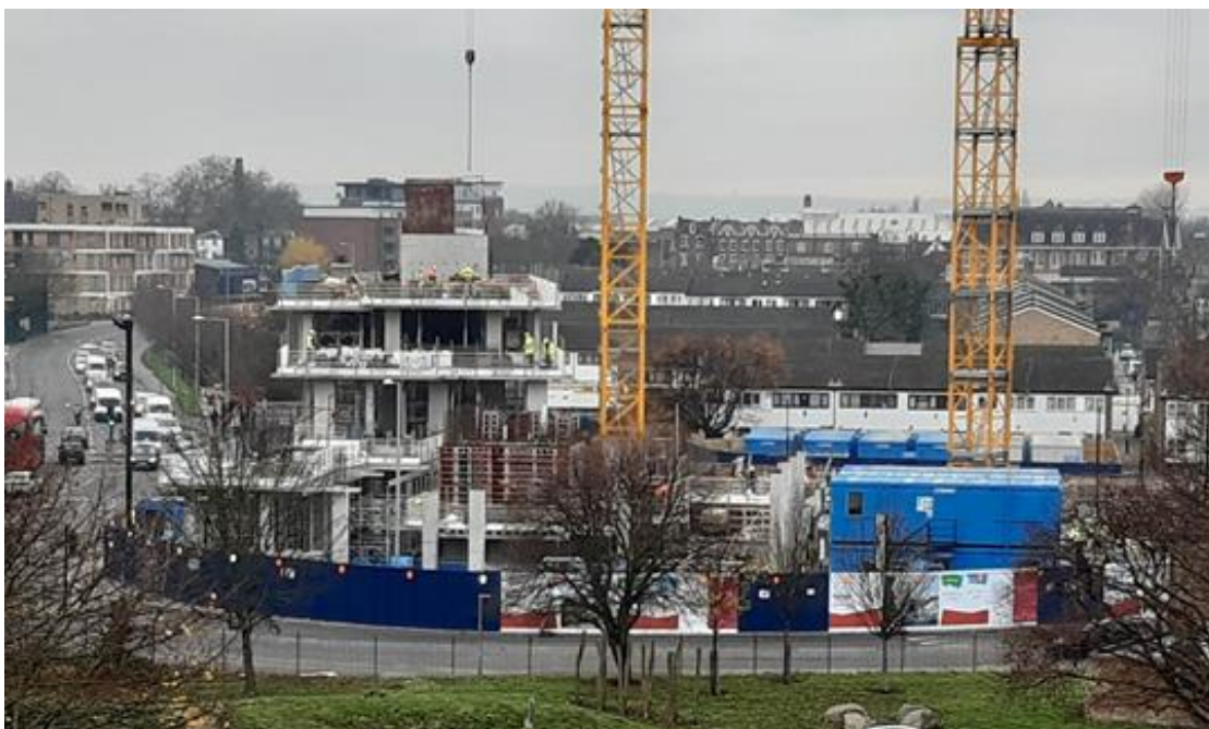
Walter Tull House, 131 Council homes for Council rent and a health centre in Tottenham Green completing June 2022
