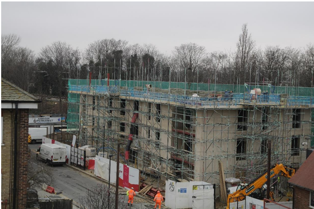
Work on Joy Gardner House , eleven Council homes for Council rent in Seven Sisters completing April 2021
