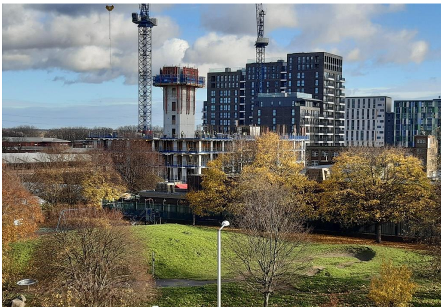
Work on Rosa Luxemburg Apartments, 102 Council homes in Tottenham Hale completing March 2022
